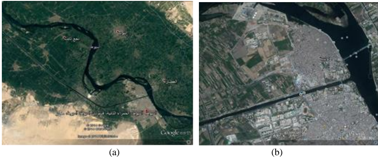
Figure 3: (a,b) show the outlet of the Ibrahimia canal at Assiut city from River Nile
