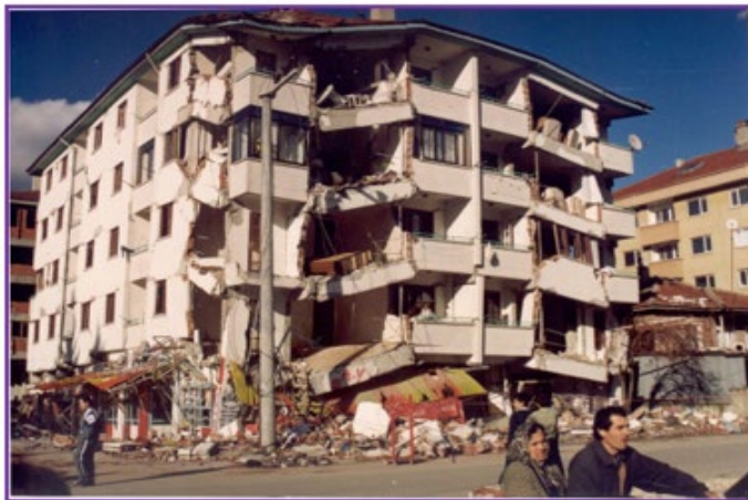
Figure 4 Bolu after the 12 November 1999 earthquake (Bolu Municipality Archive)
