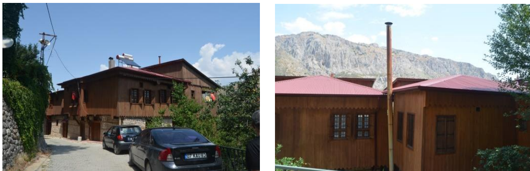
Figure 10: Contribution of traditional building to street silhouette in Erzincan-Kemaliye, cladding with local materials
