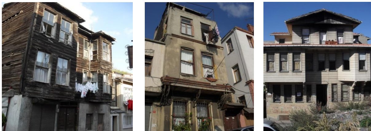
Figure 3: Planning of the buildings in the historical peninsula of Istanbul with reference to the prevailing wind and sun use
