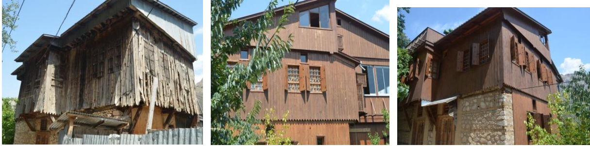
Figure 11: Facade cladding decisions and material selections of the building in Erzincan-Kemaliye town
