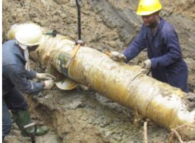
Figure 1: Technicians carrying out repair work on a vandalized pipeline.
