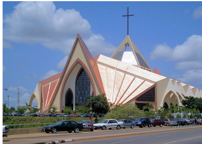
Figure 13 Exterior view - National Ecumenical Center, Abuja Source Google Photos
