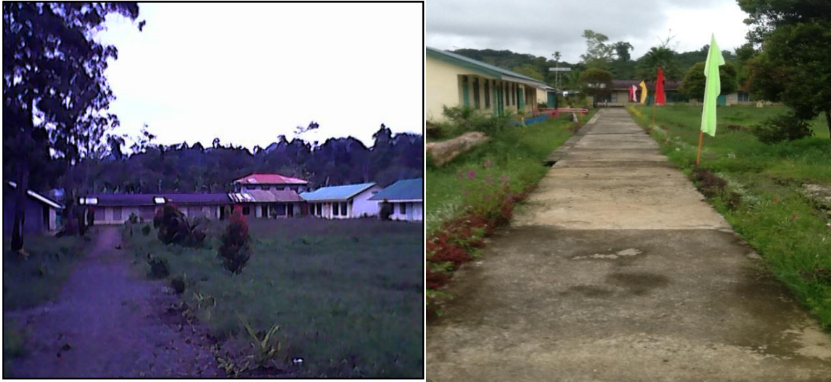
Plate No. 4: From left, the unconcreted pathway, photo taken last June, 2013, and concreted pathway, photo taken last May 2017 (Photo courtesy by the author)
