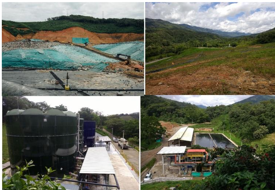
Figure 6: La Pradera landfill site showing a vase being filled and another vase after closure (up) and the lixiviate treatment plant (down) (photos taken by the author)
