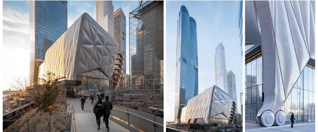
Figure 17 (a), (b), & (c) The Shed, As Seen from Different Views on Eight Bogie Wheels, The Building's Retractable Shell Rolls Out. Giovannini (2019).
