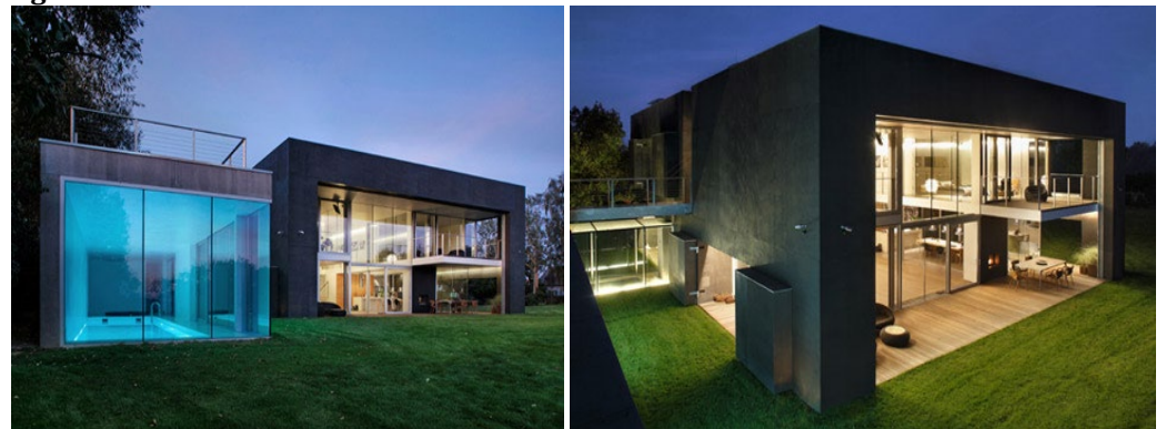
Figure 23 (a) The Building with a Swimming Pool and (b) Shows the Connected Drawbridge Frearson (2012) .
