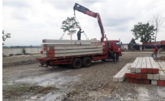
Figure 2 Bring in the Materials of Pile Foundation
