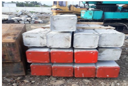
Figure 3 Placing Pile Foundation Materials Near the Pile Point
