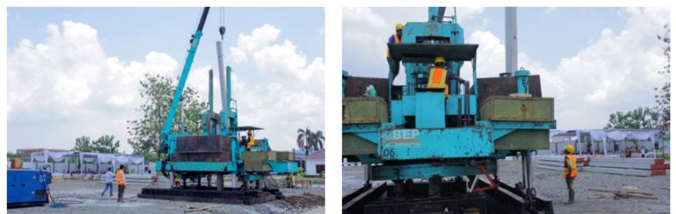
Figure 4 Setting up the Pile Foundation and Erecting Process
