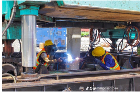
Figure 5 Welding to Splice the Pile Foundation Materials
