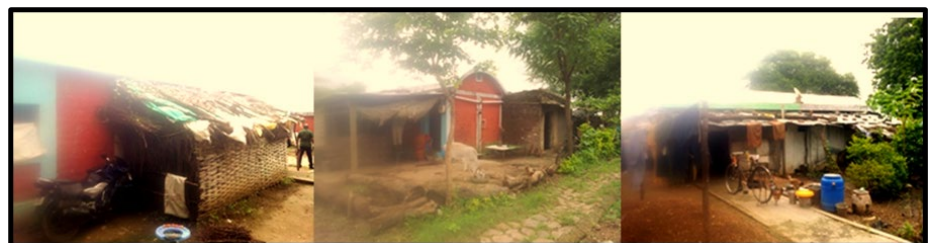
Figure 3 Extensions added to the houses in the community, Kanhapur
