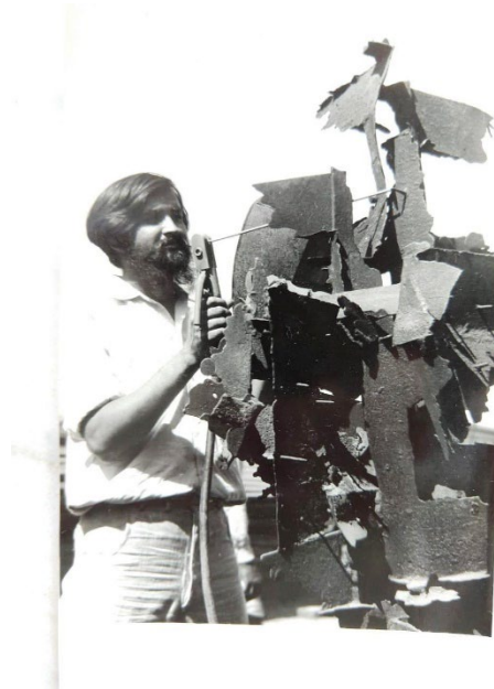
Figure 5 Kaneria welding his work
