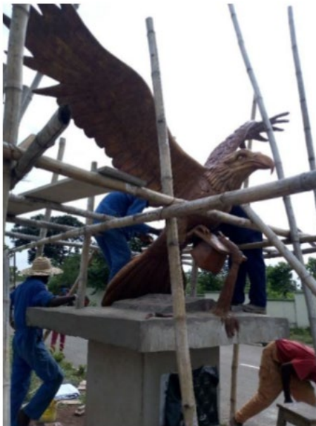
Plate 5 Improvised Scaffolds Construction Around the Conceptualised Eagle for Easy Accessibility and Proper Finishing Dimension: 275 Cm Diameter X 244 Cm High Medium: Bamboo, Cement, Sand, Mild Steel Rods, Chicken Wire and Binding Wire Year: 2021 Source: Ephraim Ugochukwu
