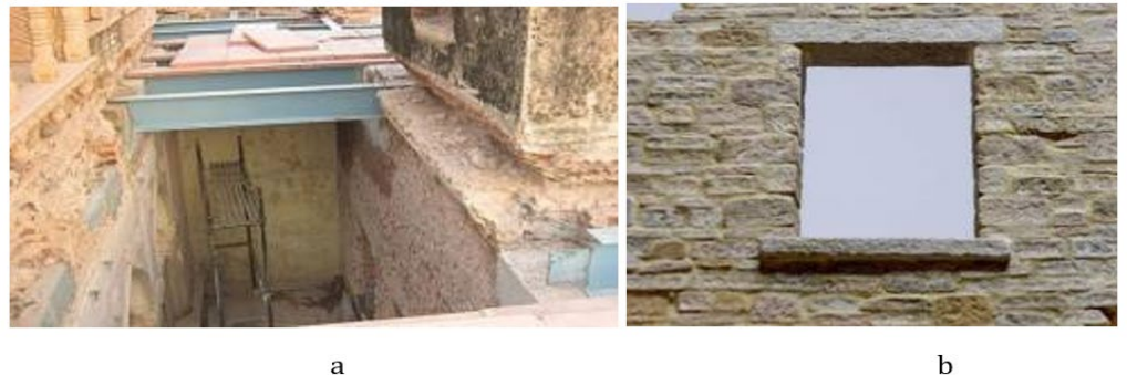
Figure 10 (a) Stone Patti Slab is Used in Place of R.C.C. slab (b) Stone Patti Lintel is Used in Place of R.C.C. Lintel.
