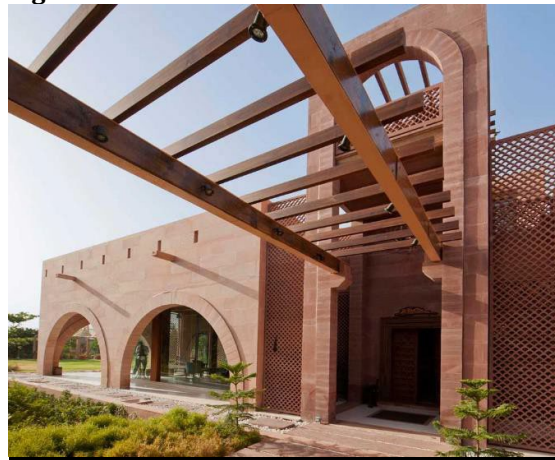
Figure 21 Use of Pergolas and Jaalis in Shunyam House Jodhpur.
