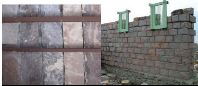
Figure 11 The Roof of a Stone Patti Arrangement (on the left) and Dressed Stone Masonry (on the Right).
