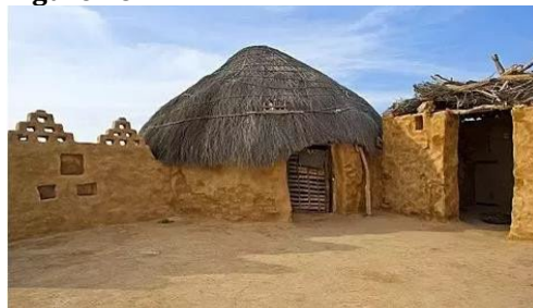
Figure 16 Traditional Rural Houses Mud Construction
