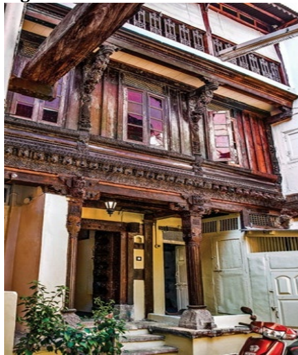
Figure 36 Front Façade of Dodhiya Haveli Source Betterinteriors.in
