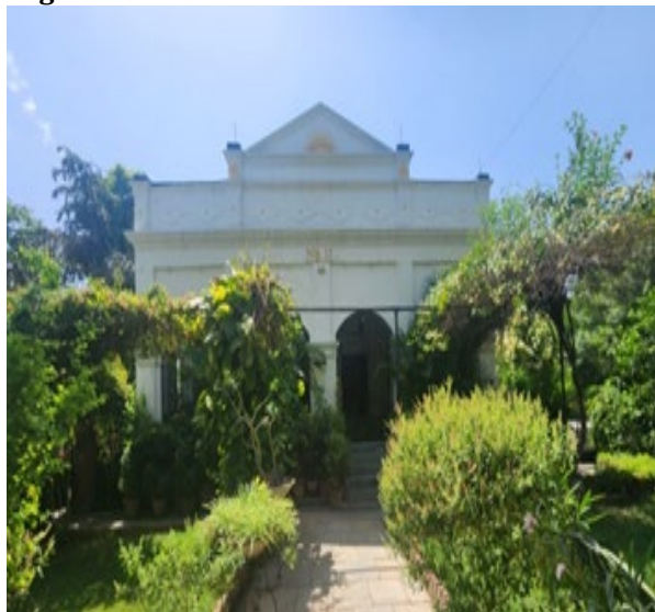
Figure 25 Front Façade of Parsi House
