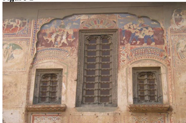
Figure 1 Current state of Navalghar Haveli-1
