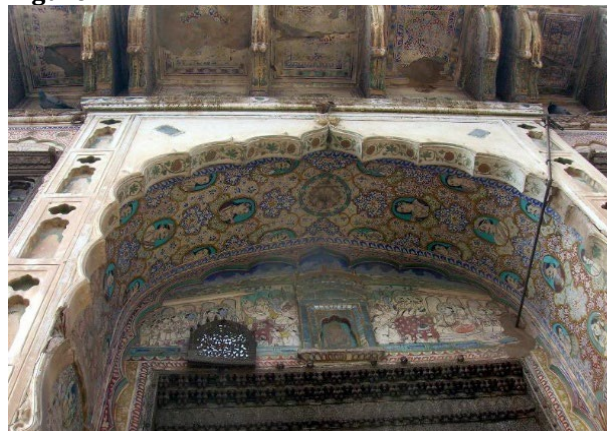
Figure 2 Current State of Navalghar Haveli - 2
