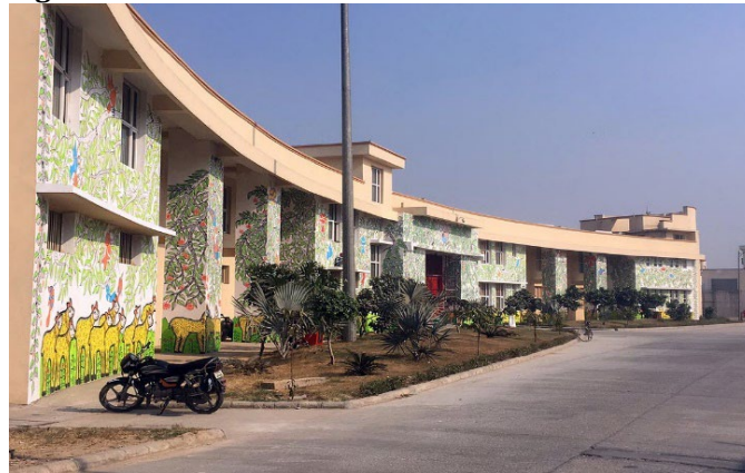
Figure 2 Exterior Walls of Mandoli Covered with Madhubani-Style Wall Art
