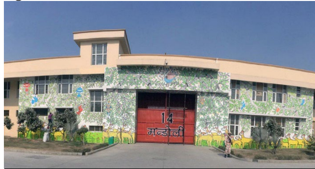
Figure 1 Mandoli Sub-Jail, Located in New Delhi, India
