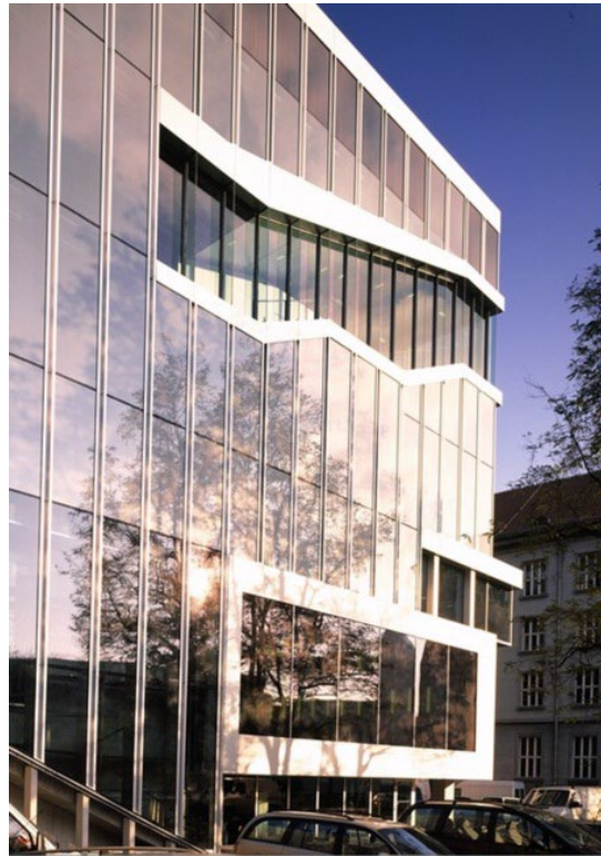
Figure 15 The Promenade's Scars on the Façade
