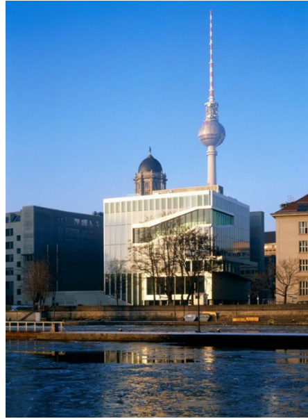
Figure 2 The Dutch Embassy and its Surroundings (2004)
