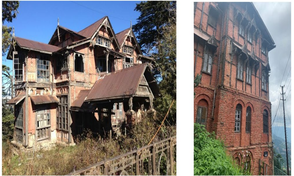
Figure 3 The Bantony Castle (Before Restoration) & Cecil Hotel in Shimla
