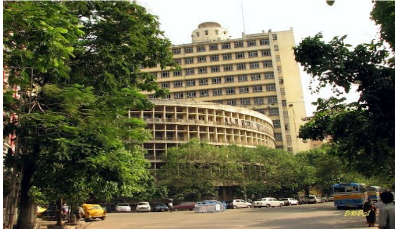
Figure 11 West Bengal's New Secretariat, Calcutta (1949-54): Juxtaposition of Geometric Forms, Vertical & Horizontal Lines
