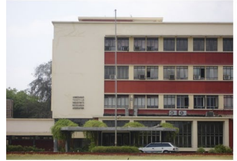
(b) The Ahmedabad Textile Industry's Research Association (ATIRA) building, Ahmedabad (1950-52)
