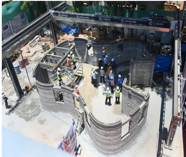
Figure 2 Construction Using 3d Printing
