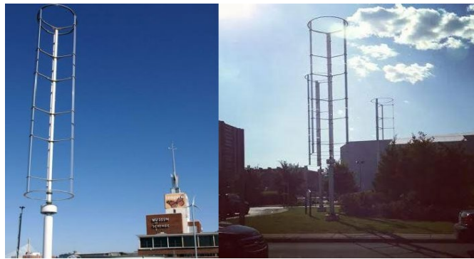
Fig 11 A vertical axis wind turbine installed at the Wind Turbines at Detroit Airport (Wind Turbines Powering Detroit Airport - green living, electric vehicle consultants, green guy, Companies, Car Expert, Electric Car News, New York, California, Florida, Missouri, Texas, Nevada (greenlivingguy.com))
